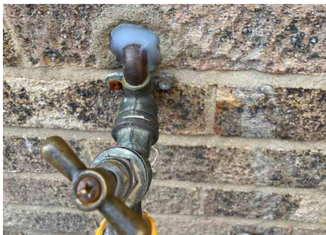
Above: Silicon seals around entry points to the property Below: Flood front door
