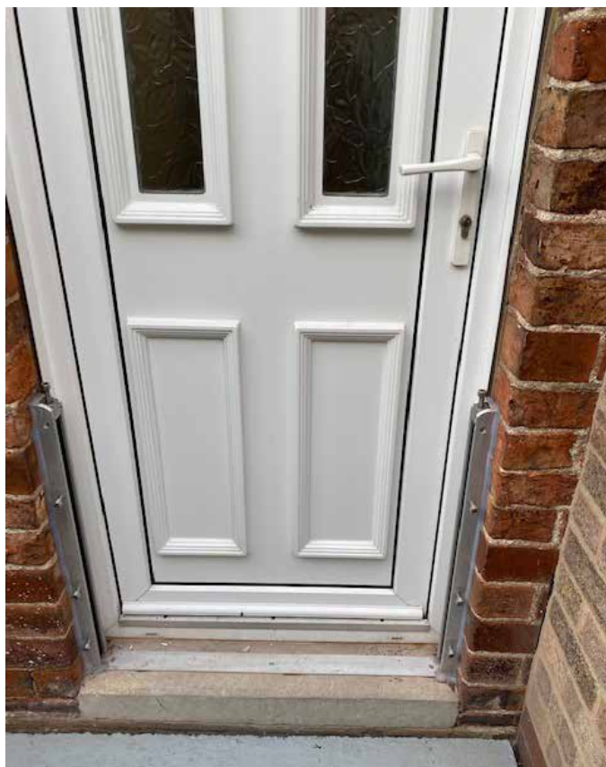
Above: Support brackets for flood barrier installed
