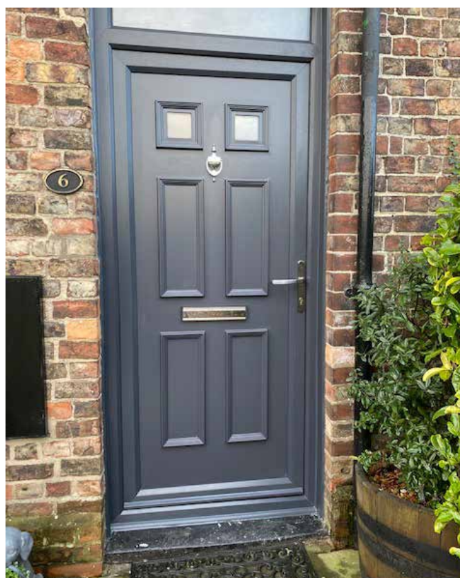
Above: Silicon seals around entry points to the property Below: Flood front door
